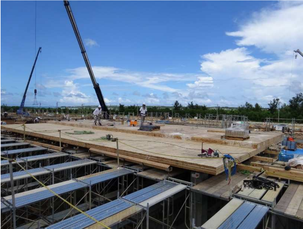
Miyako Shimojishima Terminal (under construction)
